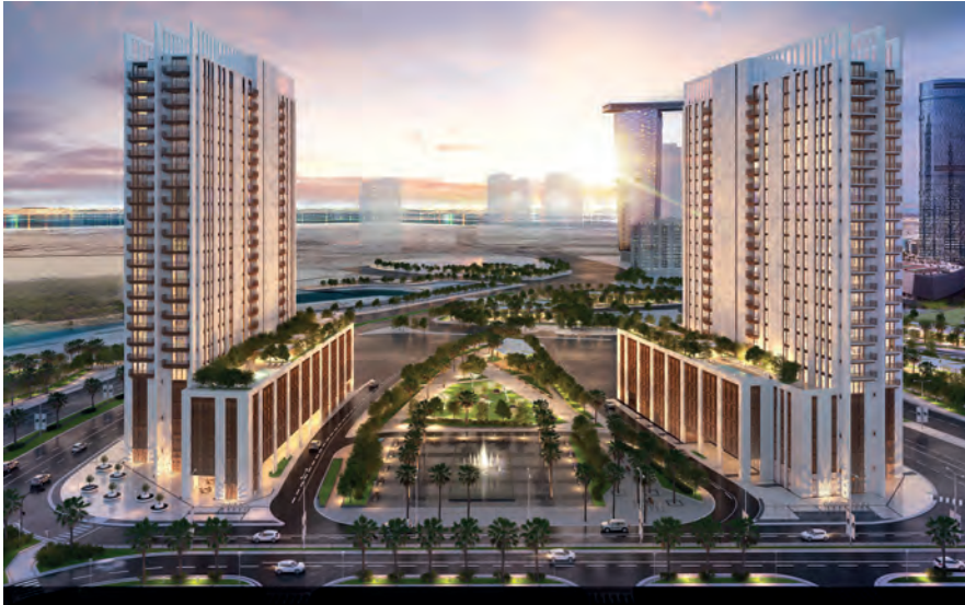
Reflection A&B Towers - Abu Dhabi
